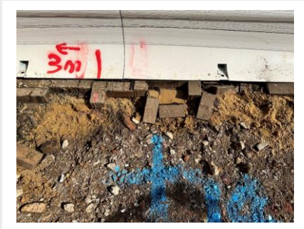
Block paviours adjacent to the piling location
