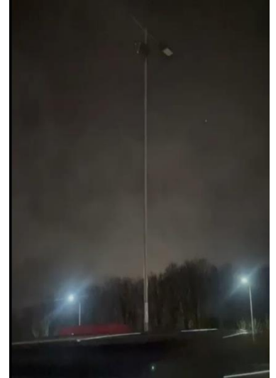
Lantern detached and hung by lanyard During Storm Henk
