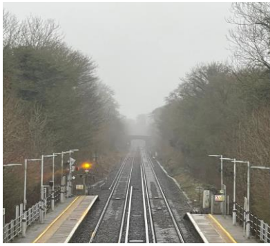
Incorrect Access Used (Down)
