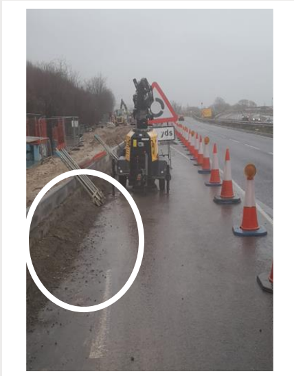
Location – Raised Kerb area
