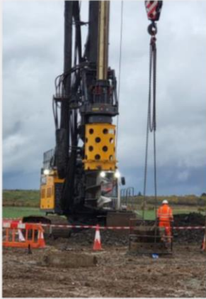
Piling rig in use at time of incident
