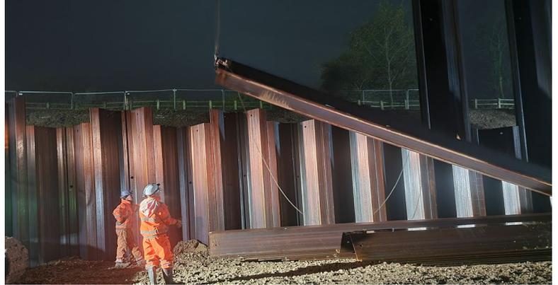
On the M25 in Potters Bar, our Highways team are well underway to stabilise an embankment which showed early signs of failing and slipping onto the main carriageway.
