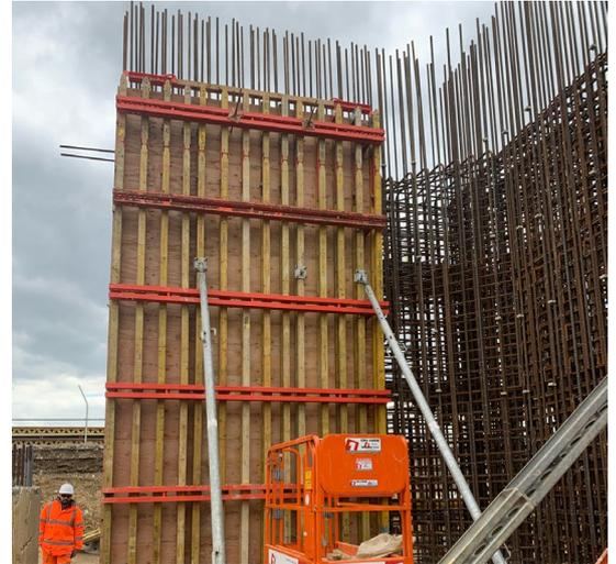
Our team at Chelmsford are making great progress constructing a new conveyor bridge for Essex County Council, which includes constructing two abutments, and have recently begun installing shutters to the formwork. Having a stable foundation is extremely important for a large project like this, to ensure our project is as successful as possible our team have been using new innovative formwork methods.
