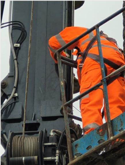
Photo showing licensed removal of nesting material working from a MEWP
