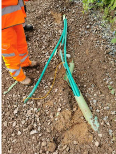
Damaged ducting.
