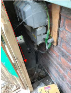
Picture 3 – Visible indication of the struck cable when the temporary door is open
