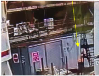
Picture 3 – Contractor office continues to rise as the Slinger Signaller is radioing to Stop. Skip detaches at this point.
