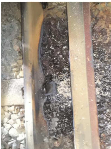
Damage to the running rail
