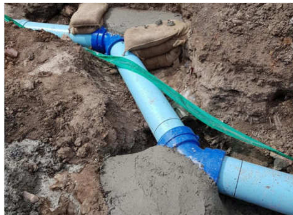
Above: Typical example of thrust block in situ.
