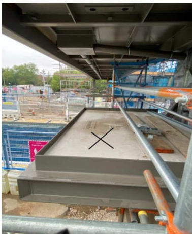
Position of Electrician on the canopy roof
