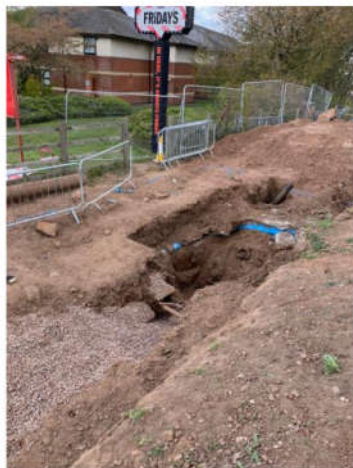
Previous Vacuum Excavation works undertaken to expose chamber location (Old watermain shown)
