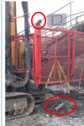
Swan neck arrangement of pipe that failed
