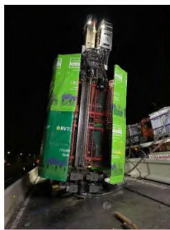
Photo of the drilling rig
