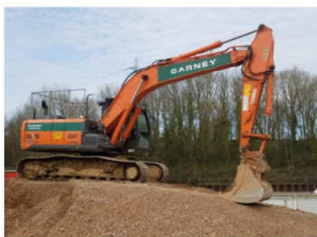
21T 360 being used to load dumper
