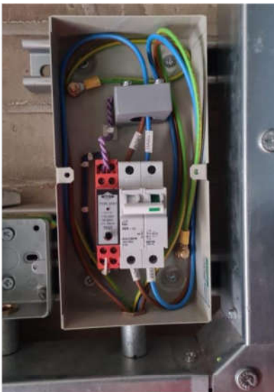
Residual Current Device (RCD) which was being worked on at time of accident
