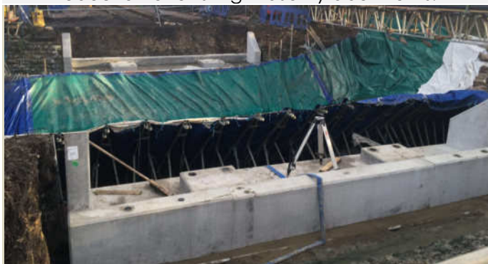
Final preparation including installation of holding dowels ready for receiving new bridge deck.
