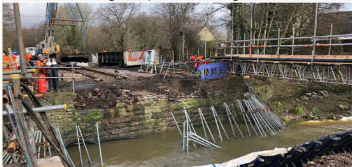
Containment of river, backfill excavation and reduction of existing masonry abutments.
