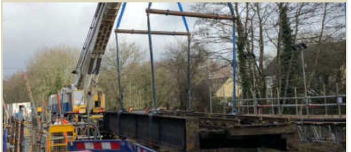
Deck removal using rail mounted crane
