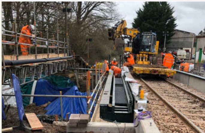
Installation of deck walkways, handrails and stairs.
