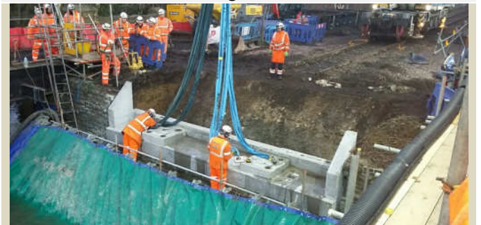
Lifting in precast concrete cill beams.
