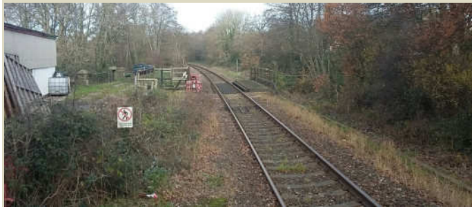
Existing 129 year old bridge deck
