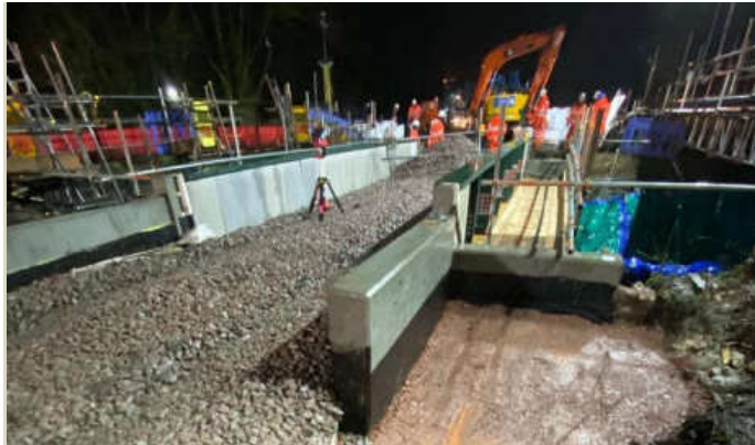
Track ballast distributed.
