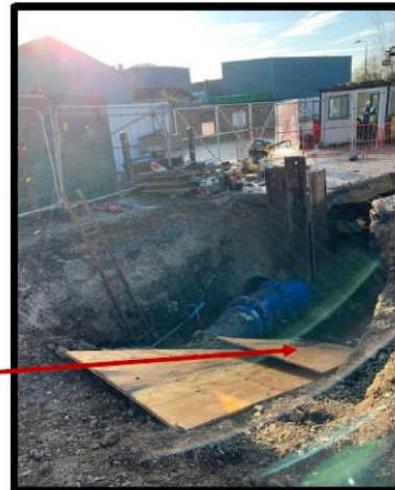
Open trench with rescue boards
