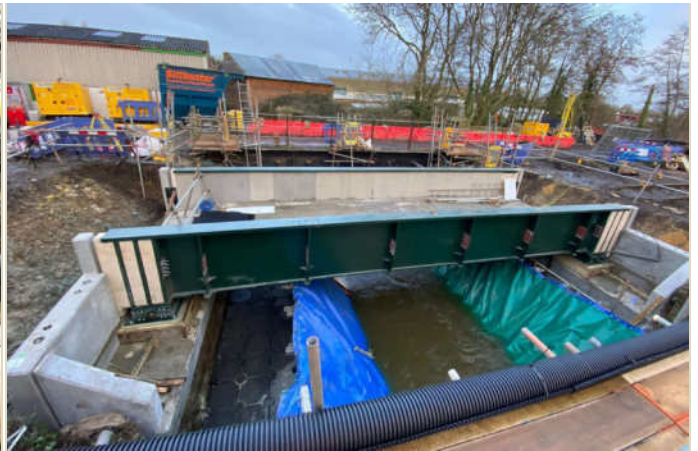
Deck lifted into final position.
