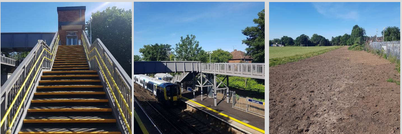
Completed footbridge, lift and link-bridge and reinstated school field.
