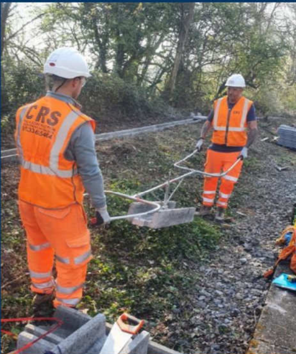
To maintain social distancing Osborne have developed an extended arm trough lifter.
