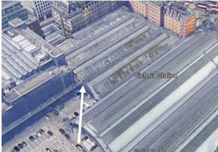
View of roof – arrow indicates location of fire
