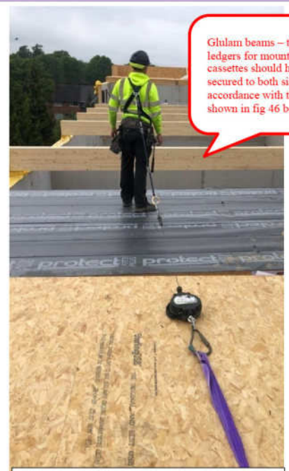
Simulation of fall arrest set up.
