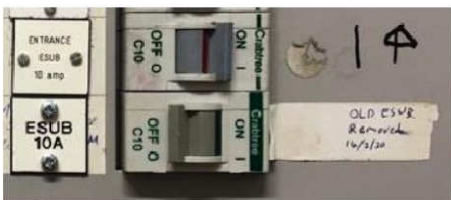
Circuit switched off & labelled at the distribution board, but not locked
