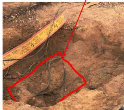
Concrete block (after removal) Approx position prior to removal
