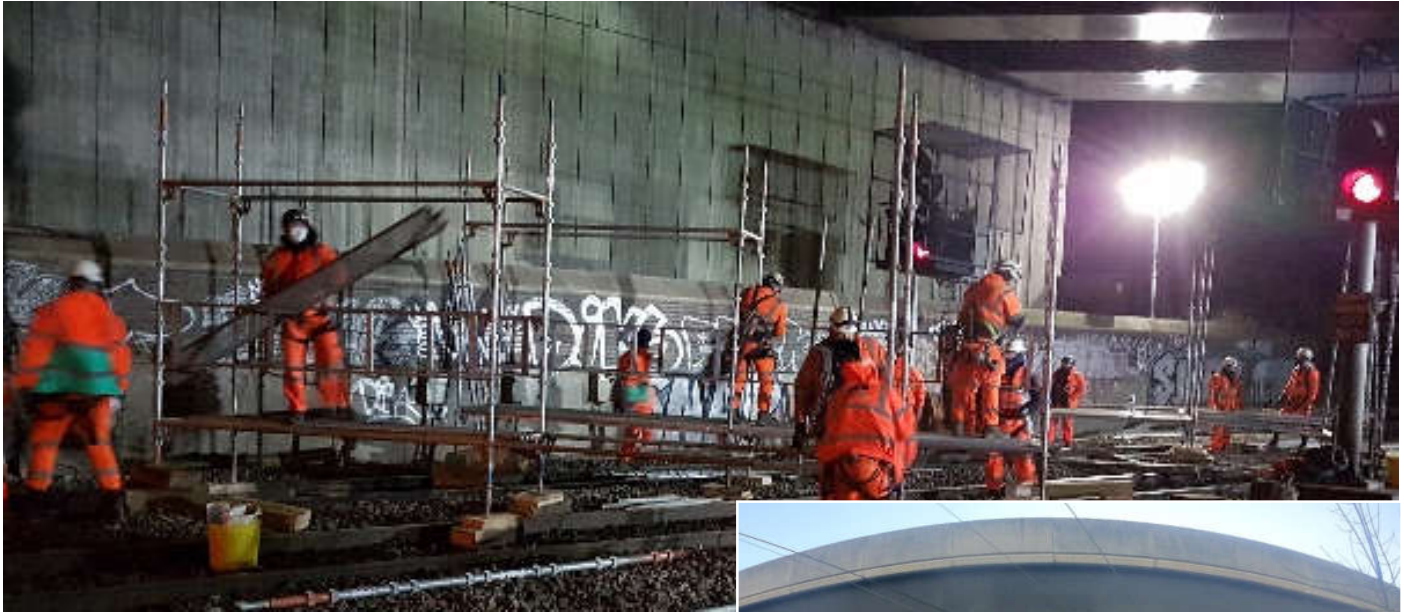
Figure – Erection of Scaffold Towers in Progress.
