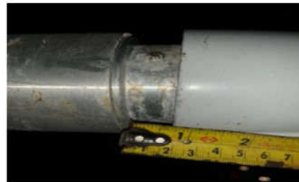
Photograph 2. Lighting Unit to Column fixing
