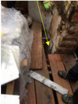
Picture 2 – How the gap was covered
