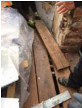
Picture 3 – infill board has now been fitted
