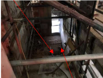
Location the operative was standing when he heard the tube falling from above. (Operative ran as soon as he heard it falling towards him).
