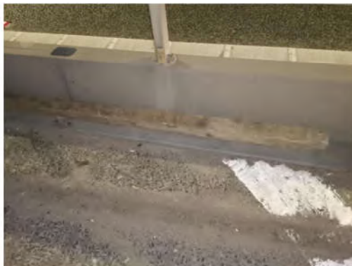
Image shows post against barrier using the flash on the
