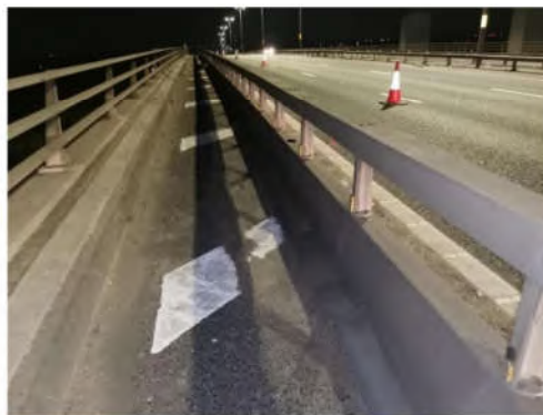
Image shows the post hidden in the shadow cast by the Streetlighting
