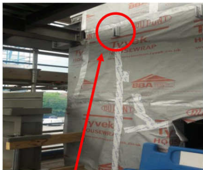
Area where Unistrut was being installed
