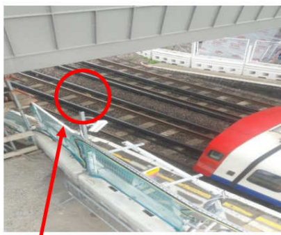
Level landed between 3 rd rail and running rail
