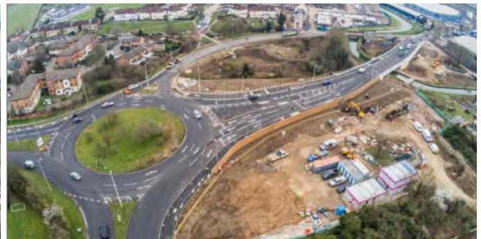
Road Open to Road Users
