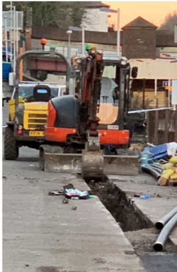
General View of trench and plant
