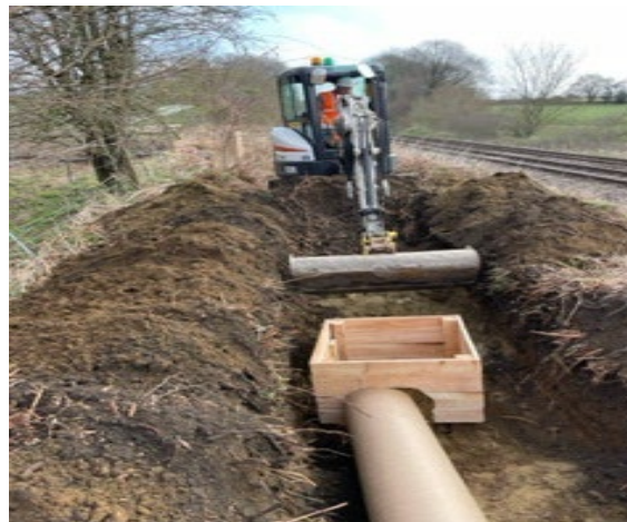
Image 1. Showing trench construction and initial sett placement
