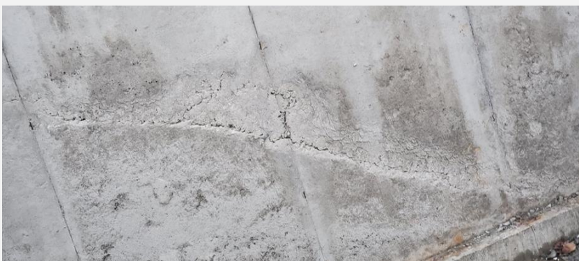
Linear cracking indicating a potential cold joint
