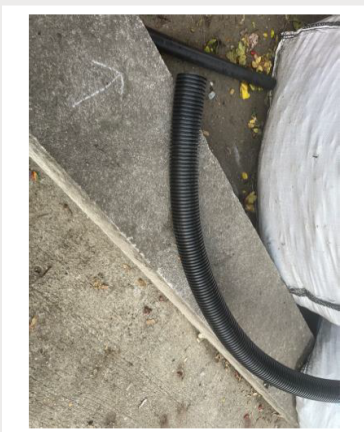
Flexible 50mm duct that was to be split along its length.
