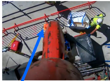
Note the slinger has stepped into the looped tagline
