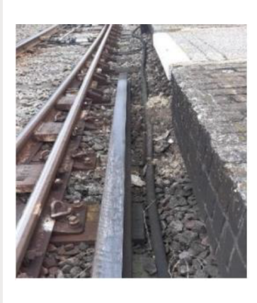
3 rd rail in cess adjacent to the platform riser wall
