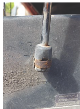
Image showing ram with retaining clip.
