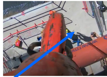
The shadow shows the slinger suspended off the ground
