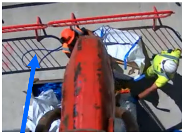
Note the blue rope tagline naturally coiling on the ground
