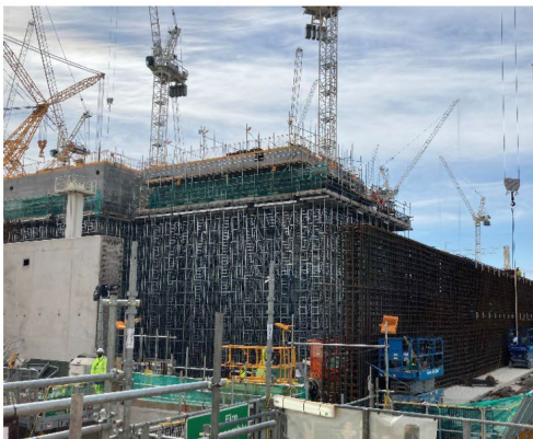
View of the CI Unit 1 Falsework
