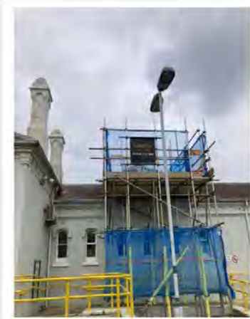
Scaffolding at Shoreham station
