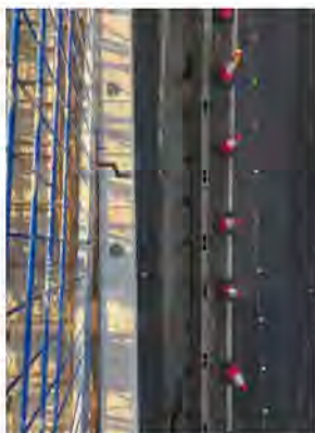
View to live carriageway below
