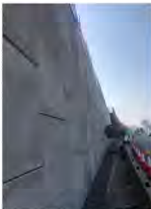
View of REW to live carriageway
