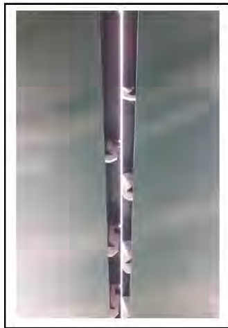
View of gap from below
