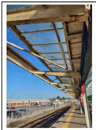
Station canopy with similar glazing panes in situ
